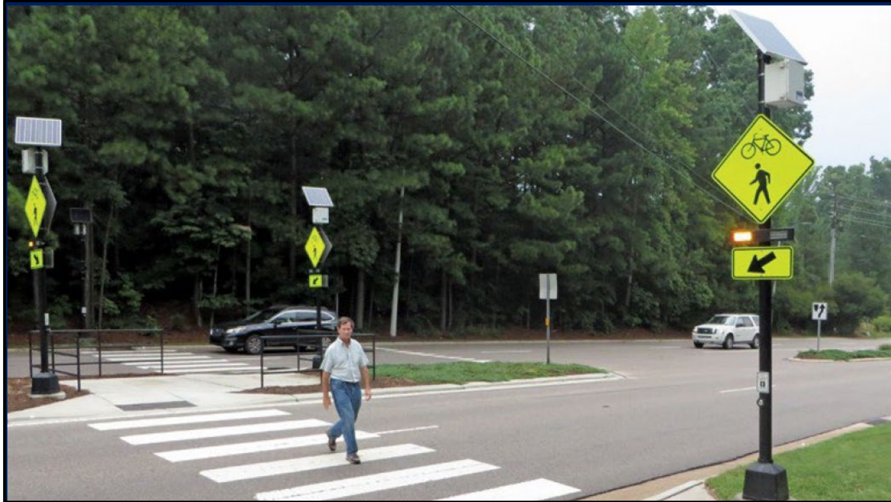
An example of a mid-block pedestrian crossing with a Rapid Rectangular Flashing Beacon (RRFB). When activated, the rapidly flashing beacons enhance the visibility of pedestrians at the crossing to motorists.
